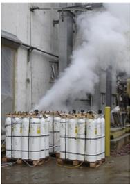
A situation that required quick action by two fumigators who donned SCBAs to close cylinder valves and secure the area. The leak was caused by a thin wall introduction line and black plastic union connectors that failed.
